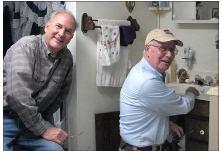
Chuck Sampson and Frank Cuthrell make repairs.
